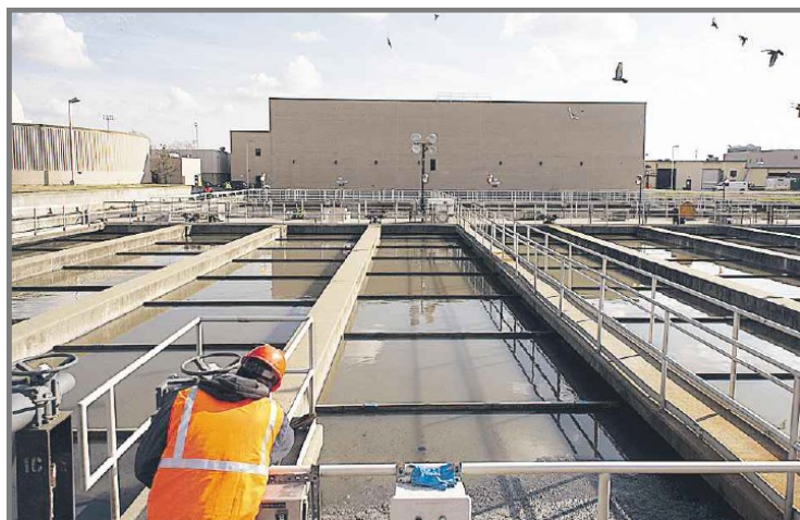
A tidal surge at the Bay Park Sewage Treatment Plant during superstorm Sandy flooded the pumping system under 9 feet of water and destroyed its electrical system.
