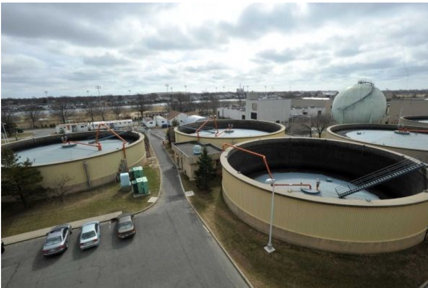
Shown are digester tanks at the Bay Park Sewage Treatment Plant in East Rockaway. At right is a 60-foot-high gas sphere on March 9, 2011. Photo Credit: Kevin P. Coughlin
